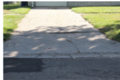
Photo 3: Cracked gutter
