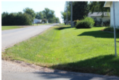
Photo 4: No curb and gutter along O Street on north and south sides
